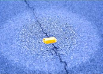
Raised pavement markers (RPMs) are small bumps, including reflectors, lining the centerline or edge line of a roadway. RPMs are often used on curves where vehicles have a higher tendency to deviate outside of the proper lane.
