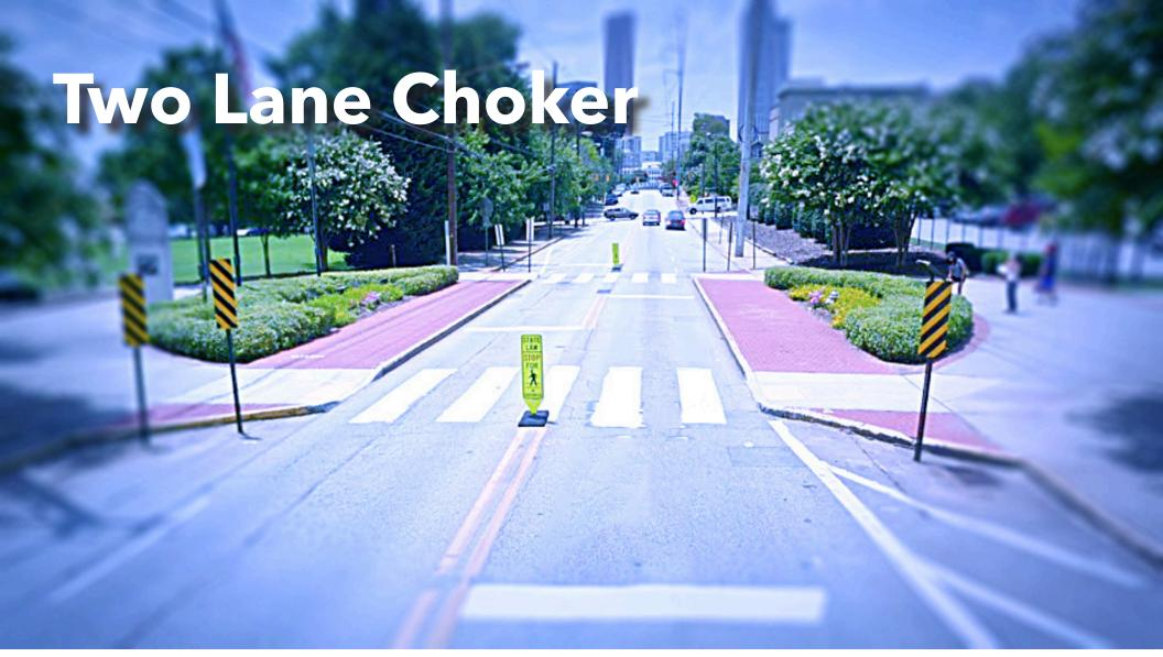
Chokers are curbing extentions at mid-block that narrow a street. Chokers leave the street cross section with two lanes that are narrower than the normal cross section which calms traffic.
