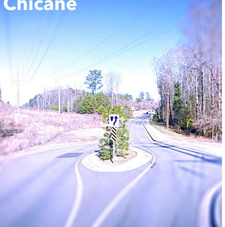
Chicanes are curb extensions that alternate from one side of the street to the other, forming S-shaped curves. The curvilinear travel pattern helps calm traffic.
