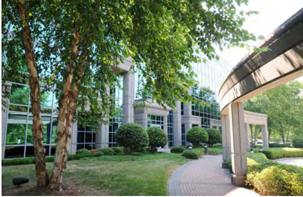
Office Complex in Johns Creek
