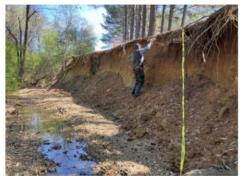
Photo 1: 10'-high eroded bank along greenway creating public safety hazard, facing upstream
