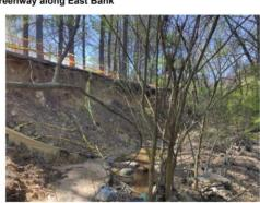
Photo 2: 10'-high eroded bank along greenway, creating public safety hazard, facing downstream
