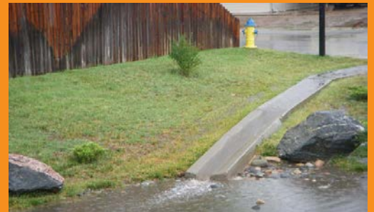
A concrete lined swale: Riprap has been added near the outlet structure to reduce velocity, allowing sediment to settle while providing erosion protection.
