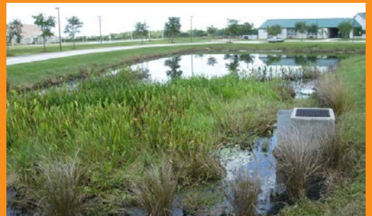
A wet detention pond provides stormwater control and an appealing amenity for residences.
