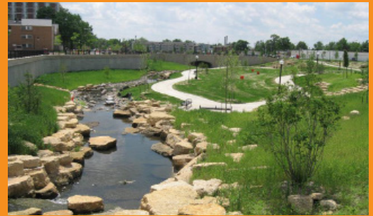
A grassy swale: riprap has been added to reduce the velocity of the runoff, allowing sediment to settle.
