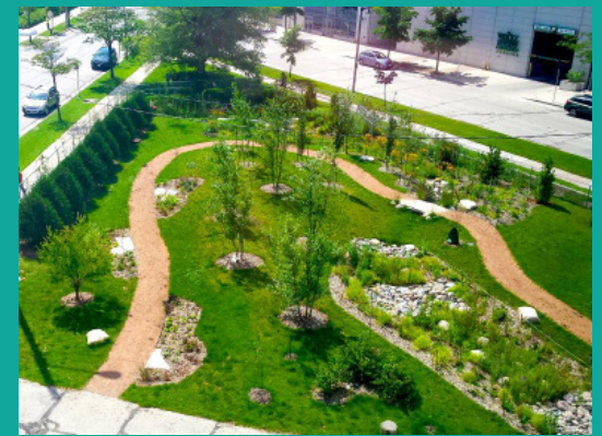
This bioretention area has an infiltration trench. The infiltration trench allows stormwater to seep into the ground during low flow conditions.
