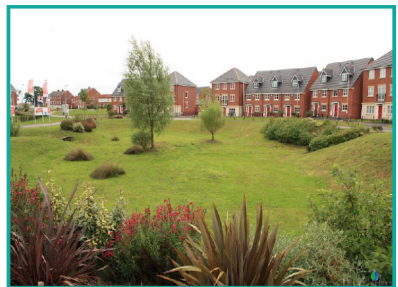
This dry detention pond contains wetland vegetation to provide additional pollution control.
