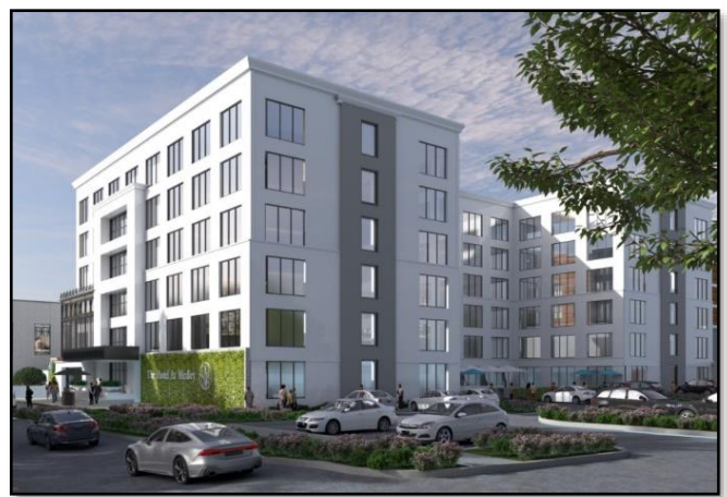
Rear View - View from Parking Lot
