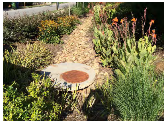
Photo 4 Linear Bioretention
