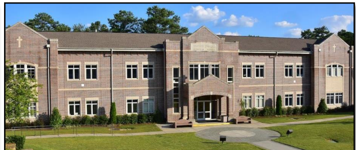
Existing School Building
